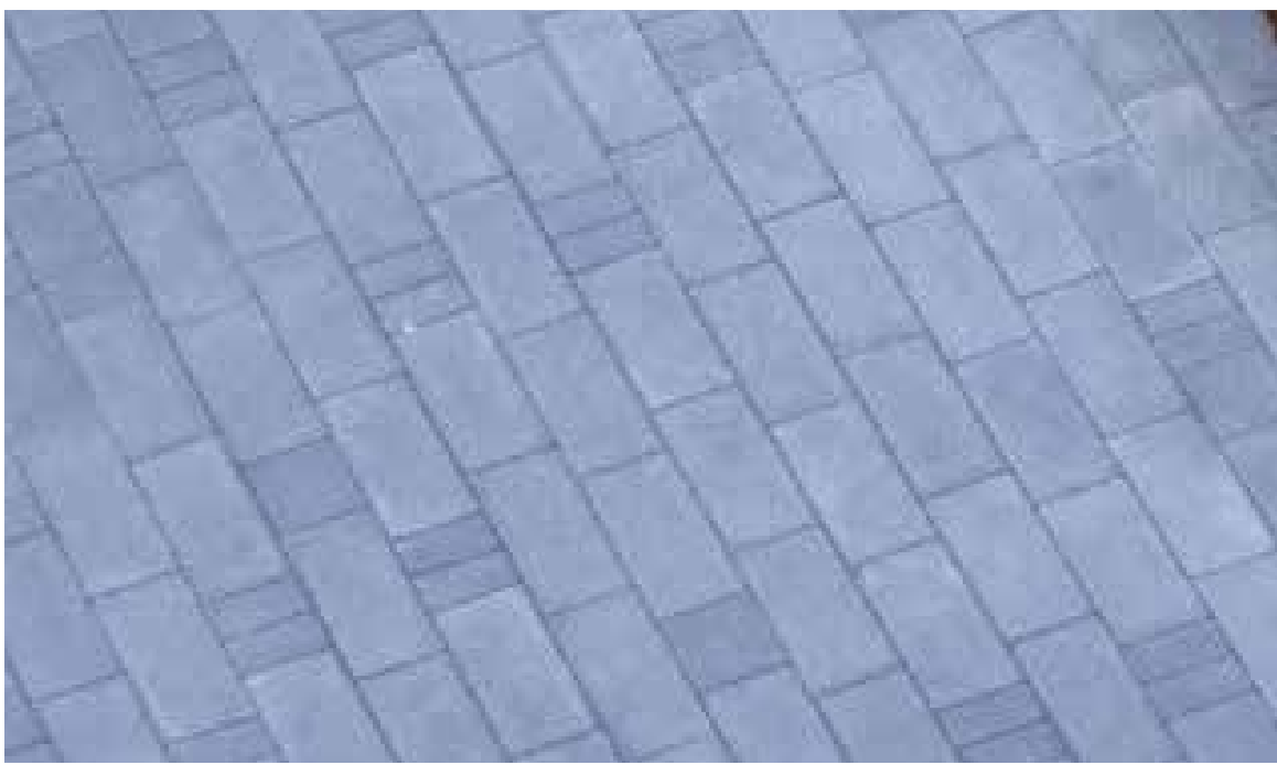
Public domain concrete feature paving
