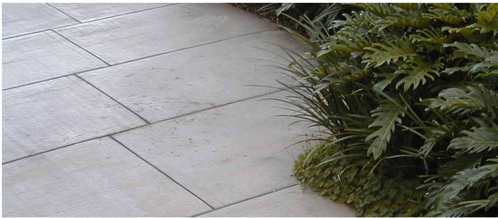
Central courtyard concrete paving
