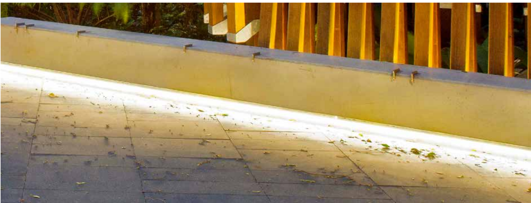
Ambient lighting along instu concrete walls
