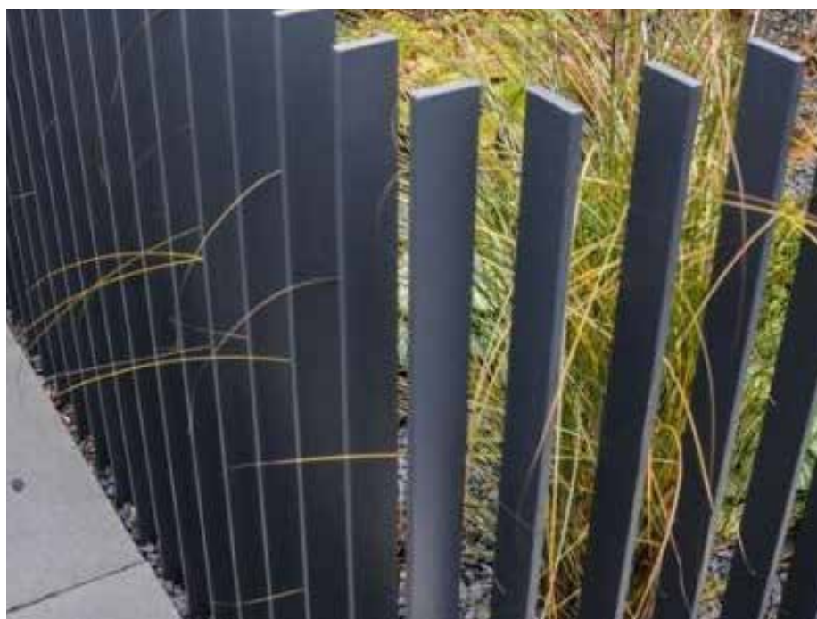
Steel balustrade to apartment terrace
