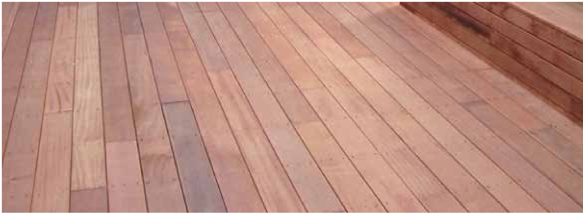
Raised timber deck
